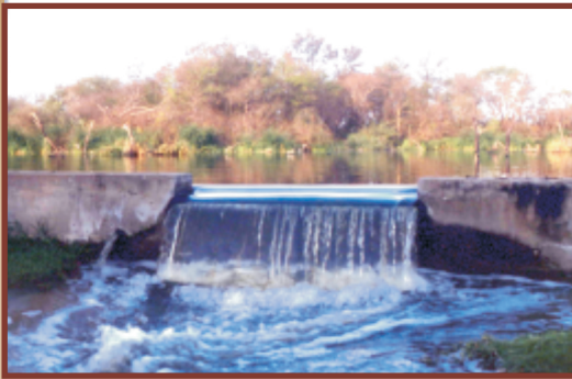
Treated wastewater discharging into the Sand River
