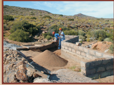
Sieving river sand for the sand filter
