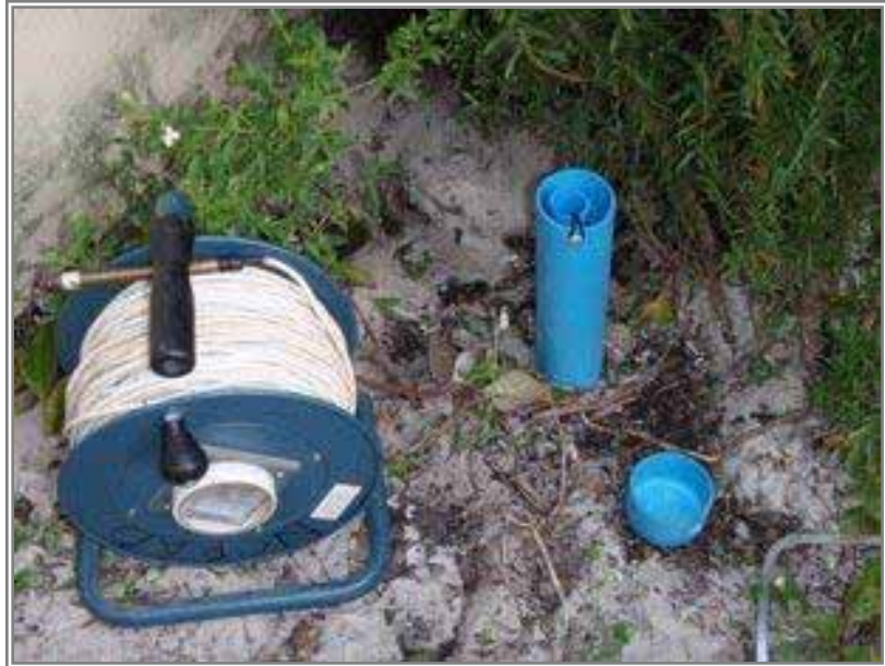
PHOTO 2 ONE OF THE TWO WELLPOINTS INSTALLED IN HERMANUS
