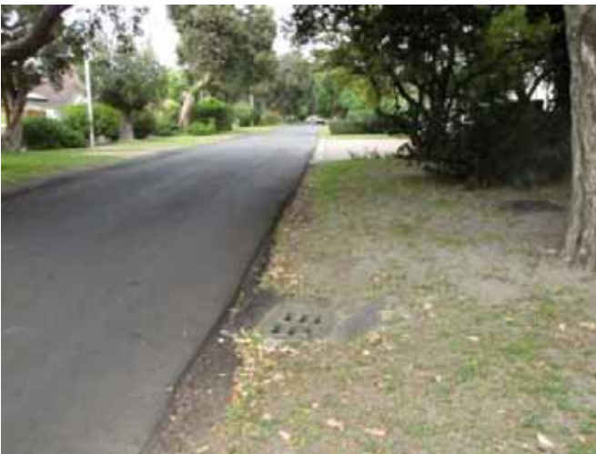
PHOTOS 4 AND 5 STORMWATER INLETS ON THE ROADS IN EASTCLIFF
