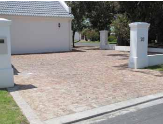
PHOTO 3 EXAMPLE OF IMPERMEABLE PAVING IN HERMANUS
