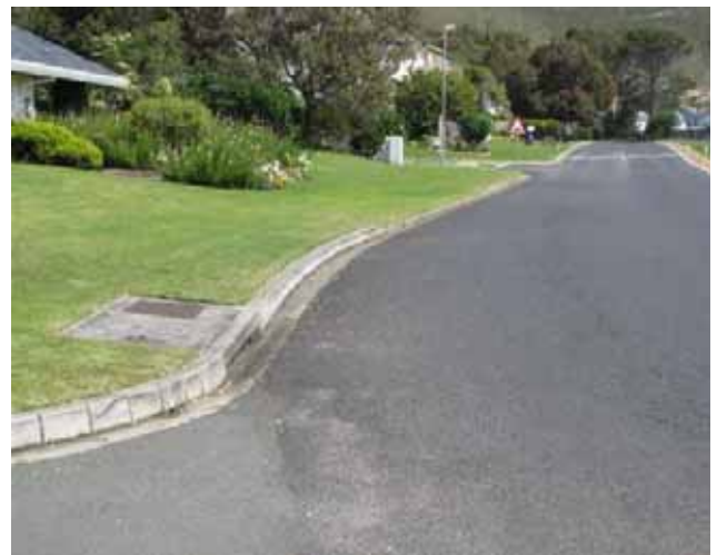
PHOTOS 4 AND 5 STORMWATER INLETS ON THE ROADS IN EASTCLIFF
